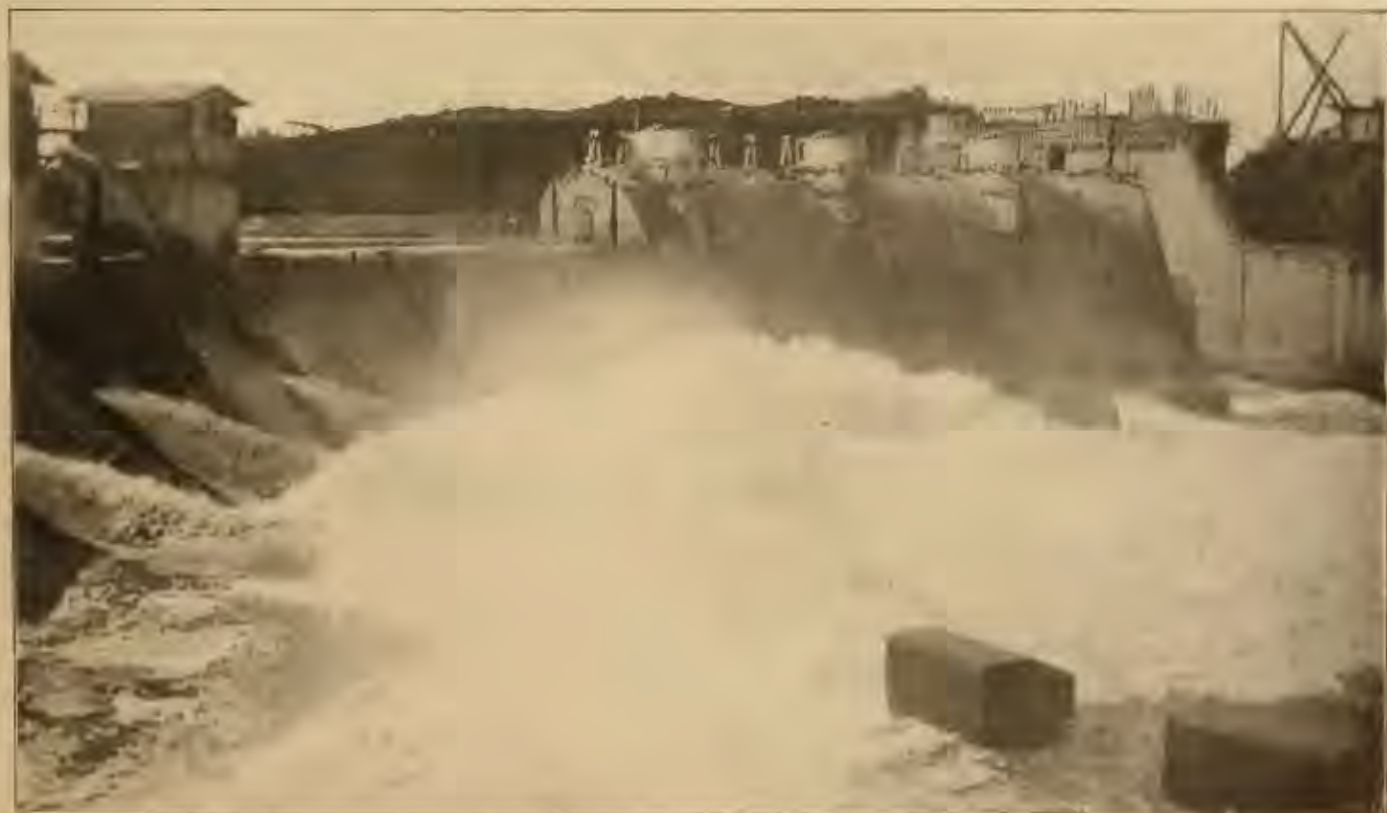
PARTLY COMPLETED SPILLWAY, 1913
