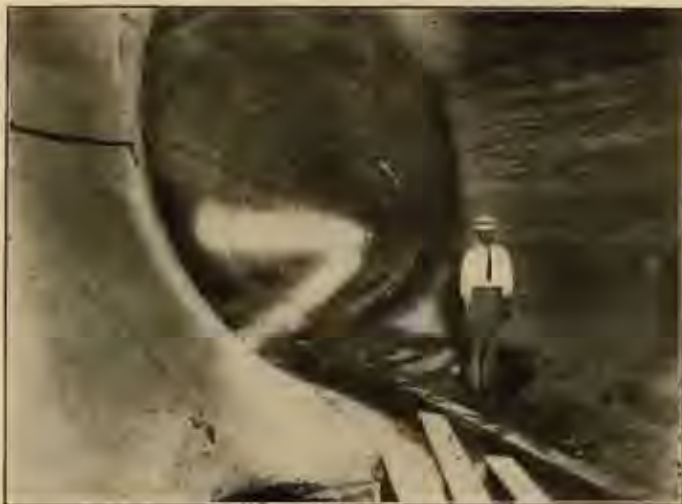
A CULVERT IN THE LOCK WALL
