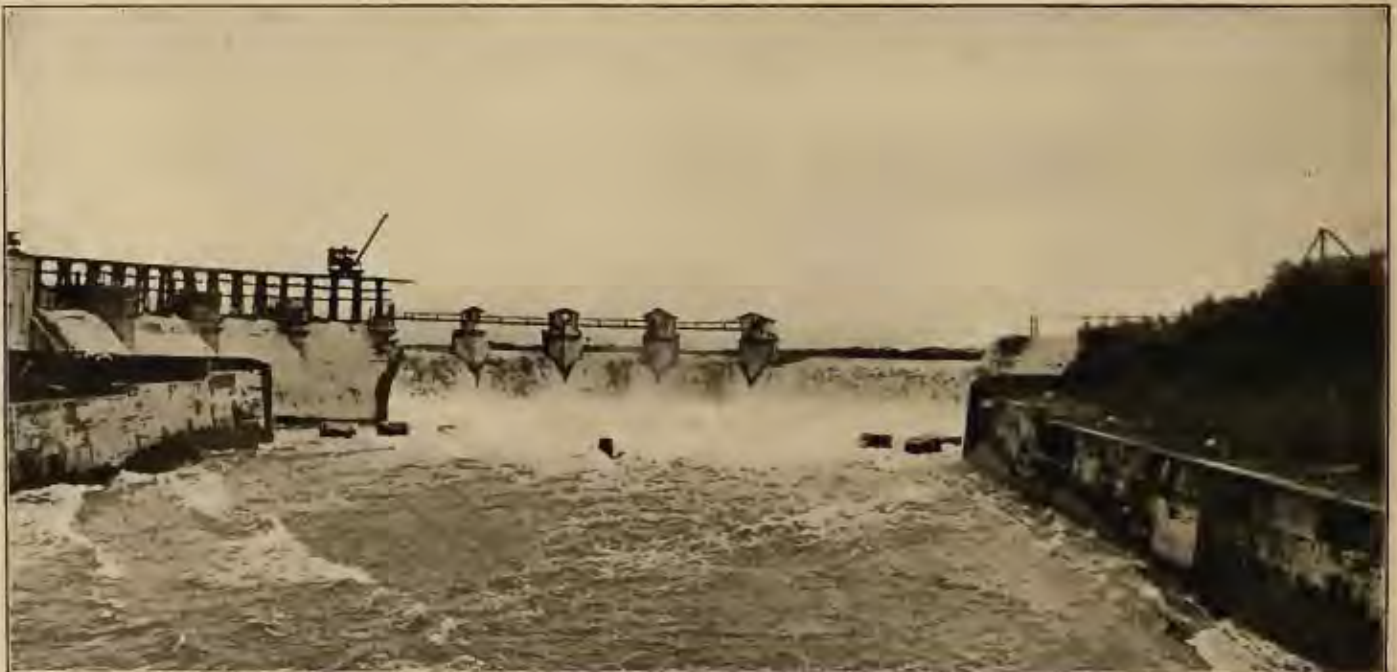
THE SPILLWAY AT HIGH WATER
