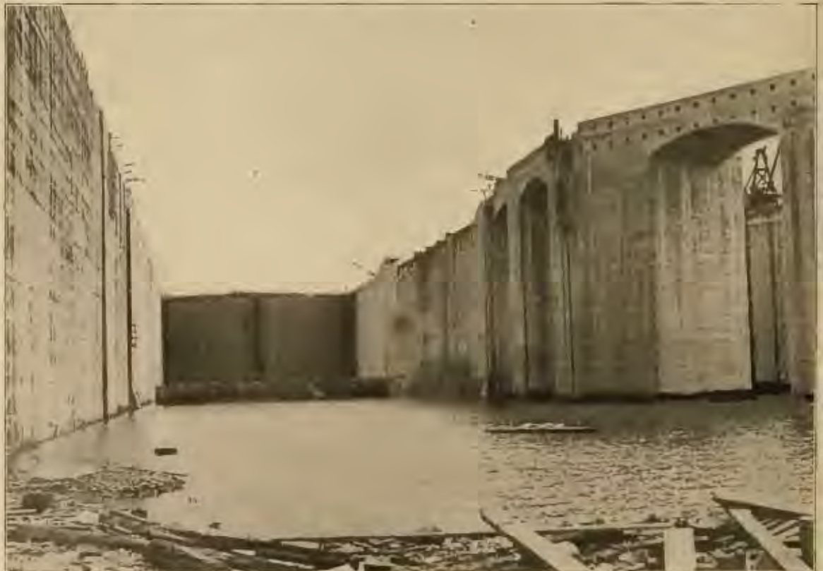
WALL OF GATUN LOCK SHOWING ARCHED CONSTRUCTION
