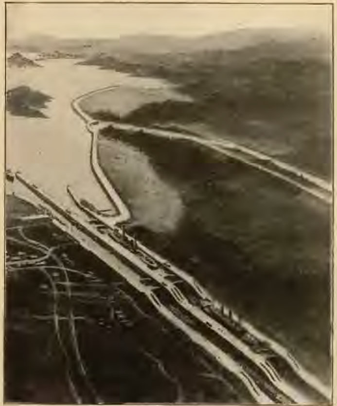
BIRD'S EYE VIEW OF GATUN DAM
