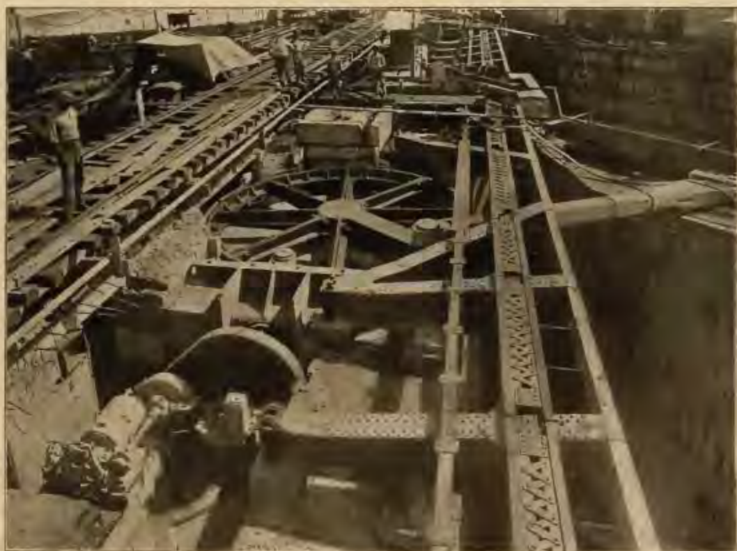
THE HEAVY WHEEL SHOWN IS THE "BULL WHEEL"
