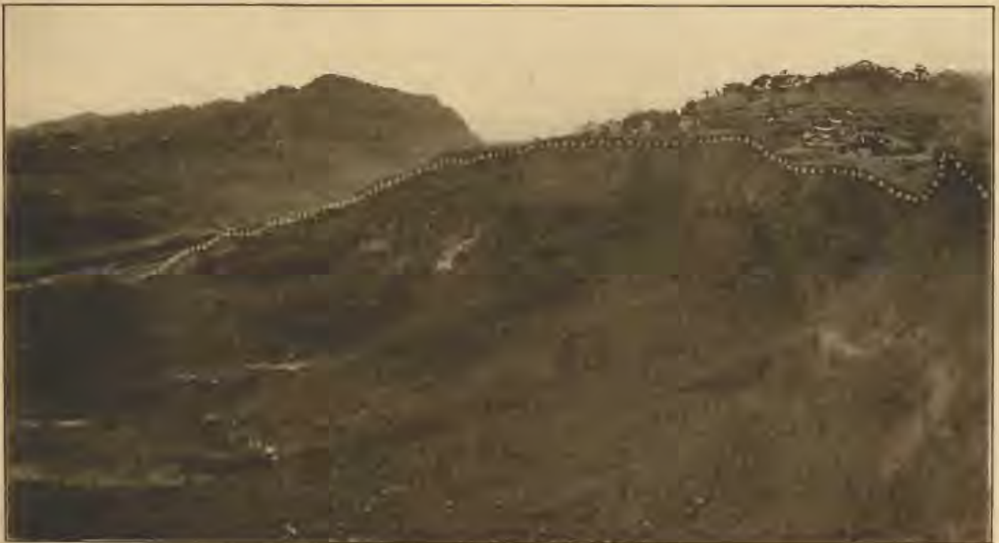
SLIDE ON WEST BANK OF THE CANAL NEAR CULEBRA
