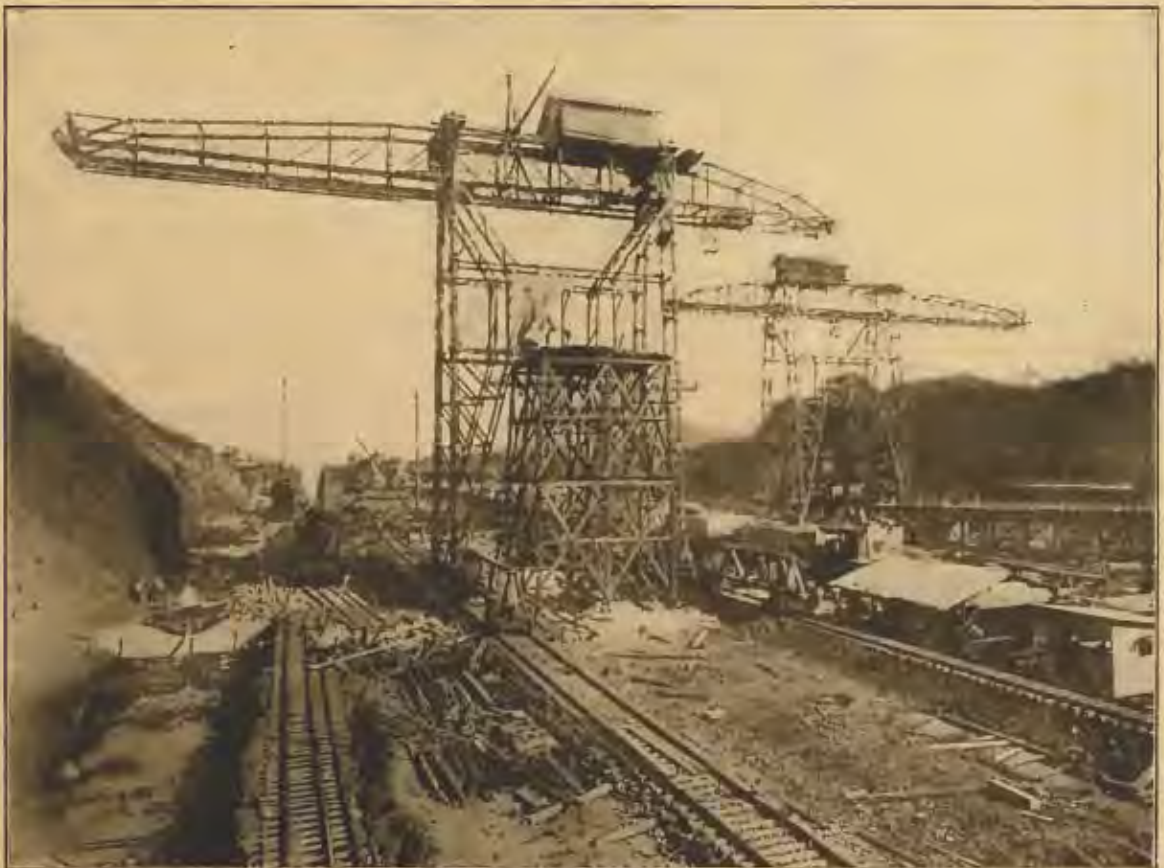
TRAVELING CRANES THAT BEAR THE BRUNT OF BURDEN CARRYING
