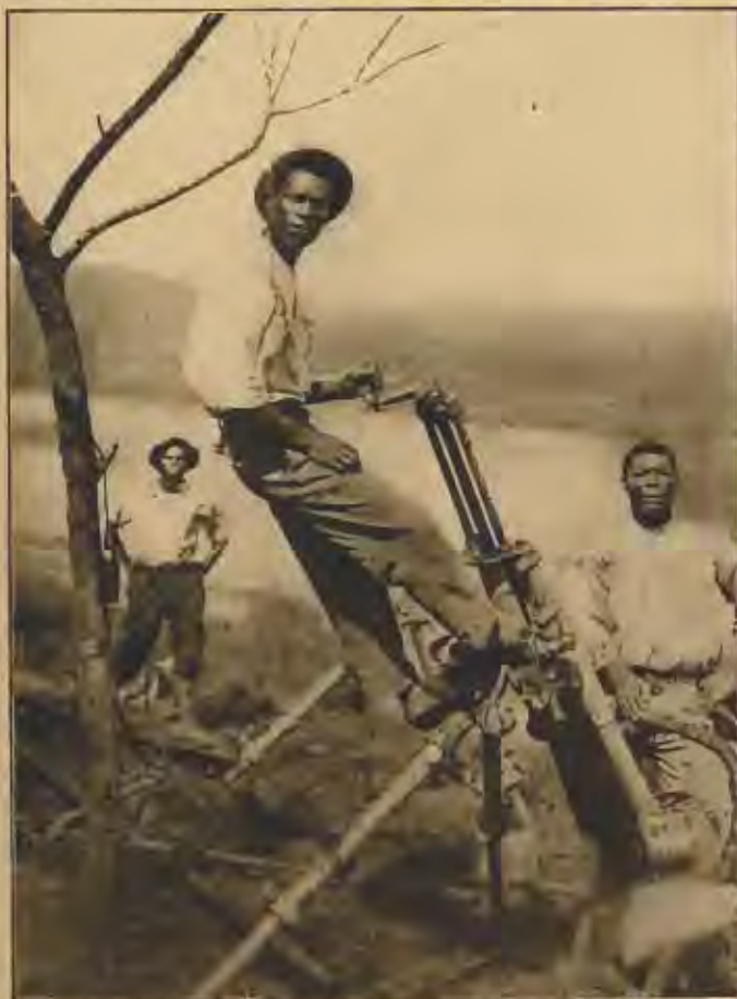
JAMAICANS OPERATING A COMPRESSED AIR DRILL
