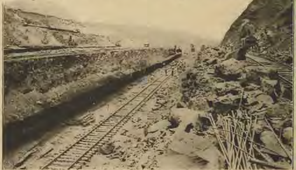
CUTTING AT BASE OF CONTRACTORS HILL
