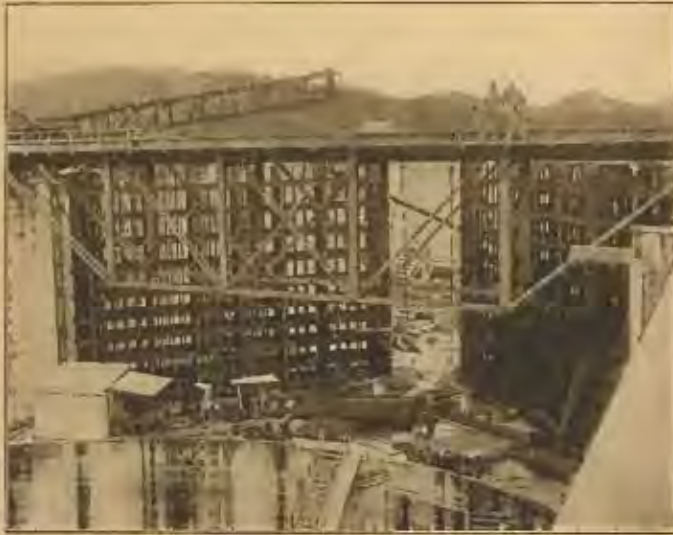
BUILDING AN UPPER TIER OF LOCKS
