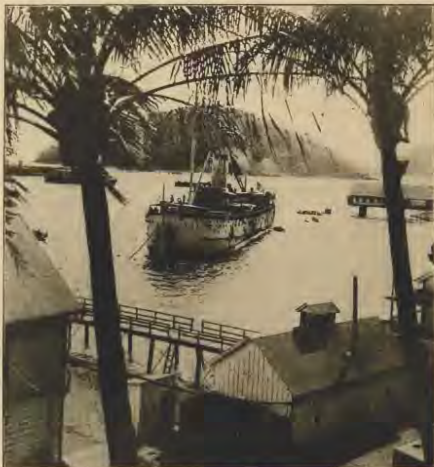
DEEP SEA DREDGE AT BALBOA
