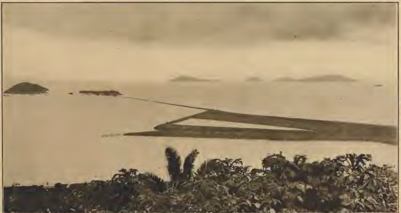
THE GREAT FILL AT BALBOA WHERE THE CULEBRA SPOIL IS DUMPED
