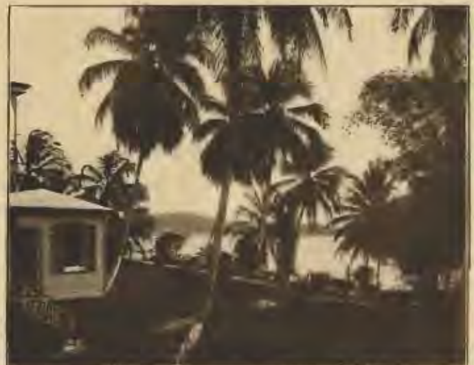
SANITARY OFFICE, BOCAS DEL TORO
