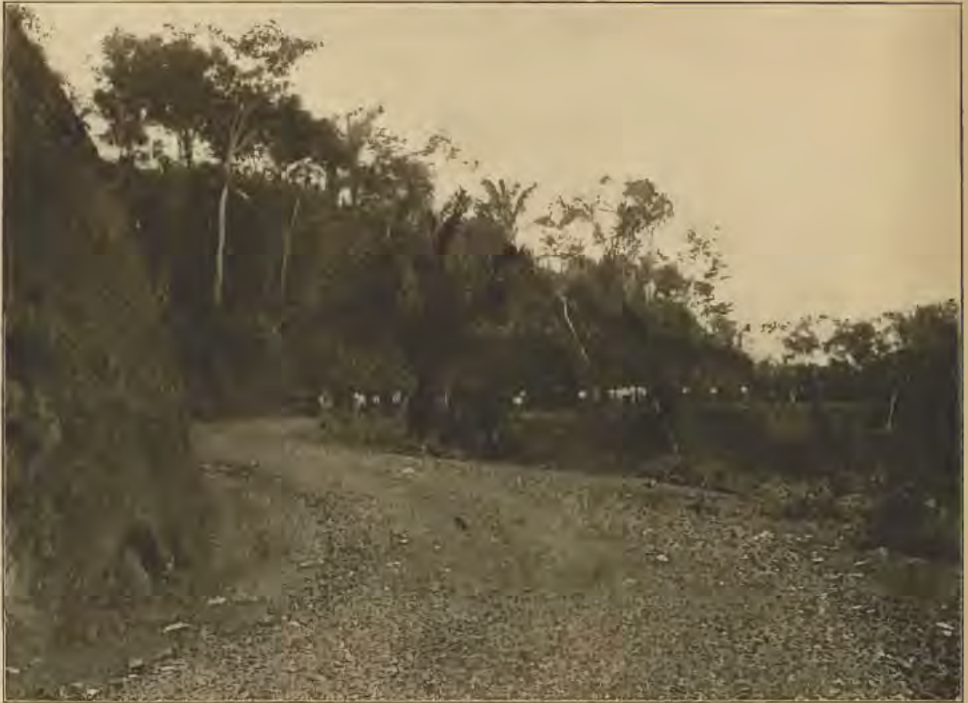
CONVICTS BUILDING A COMMISSION ROAD
