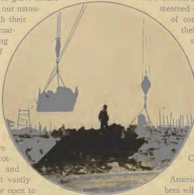
HANDLING BROKEN ROCK
