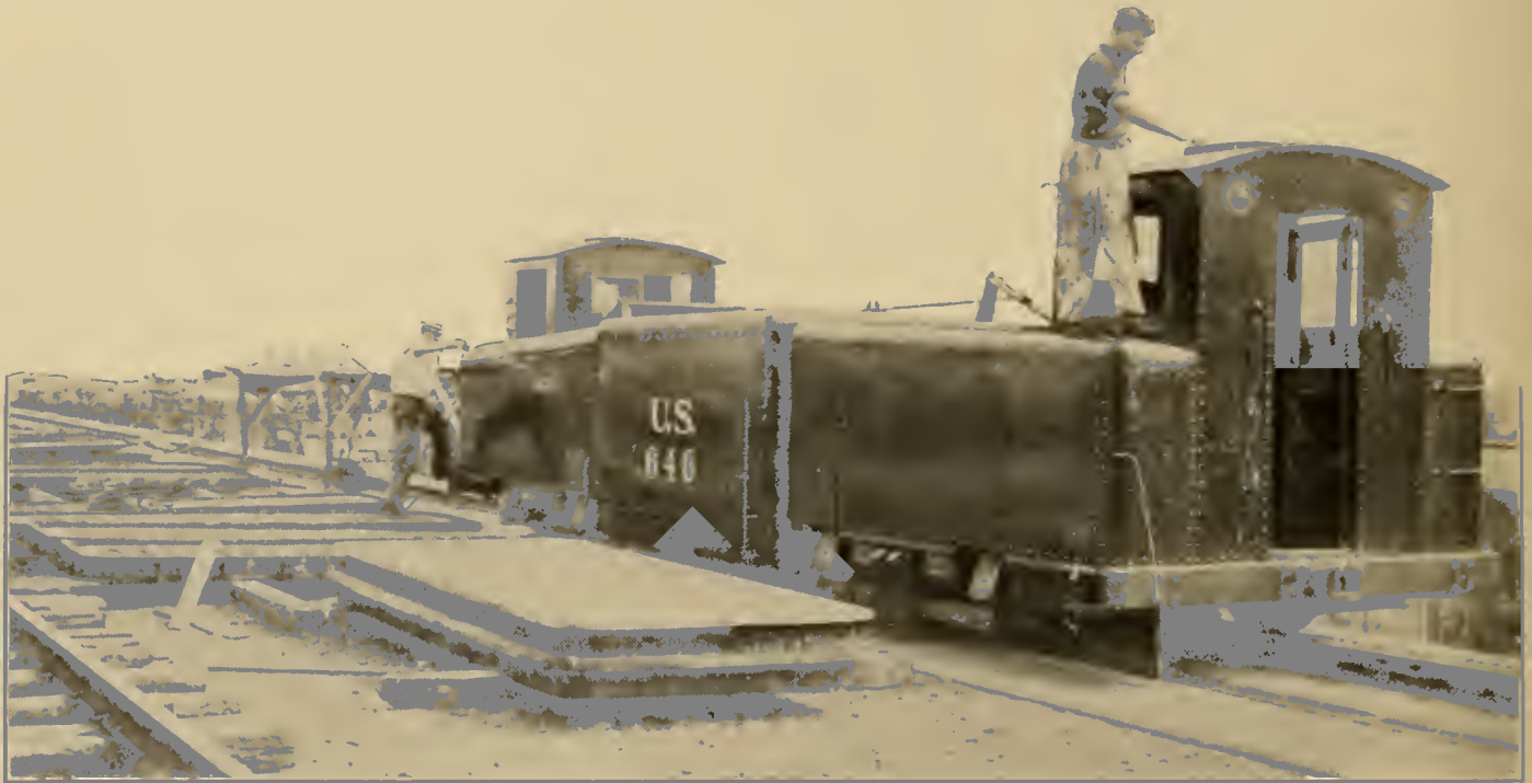
ELECTRIC TOWING LOCOMOTIVES ON A LOCK
