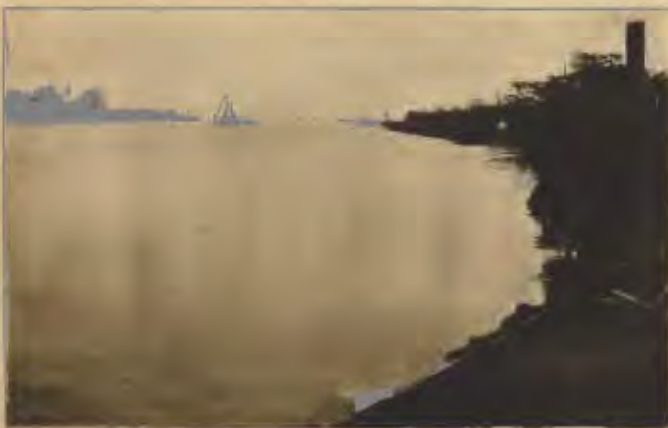
PART OF THE COMPLETED CANAL
