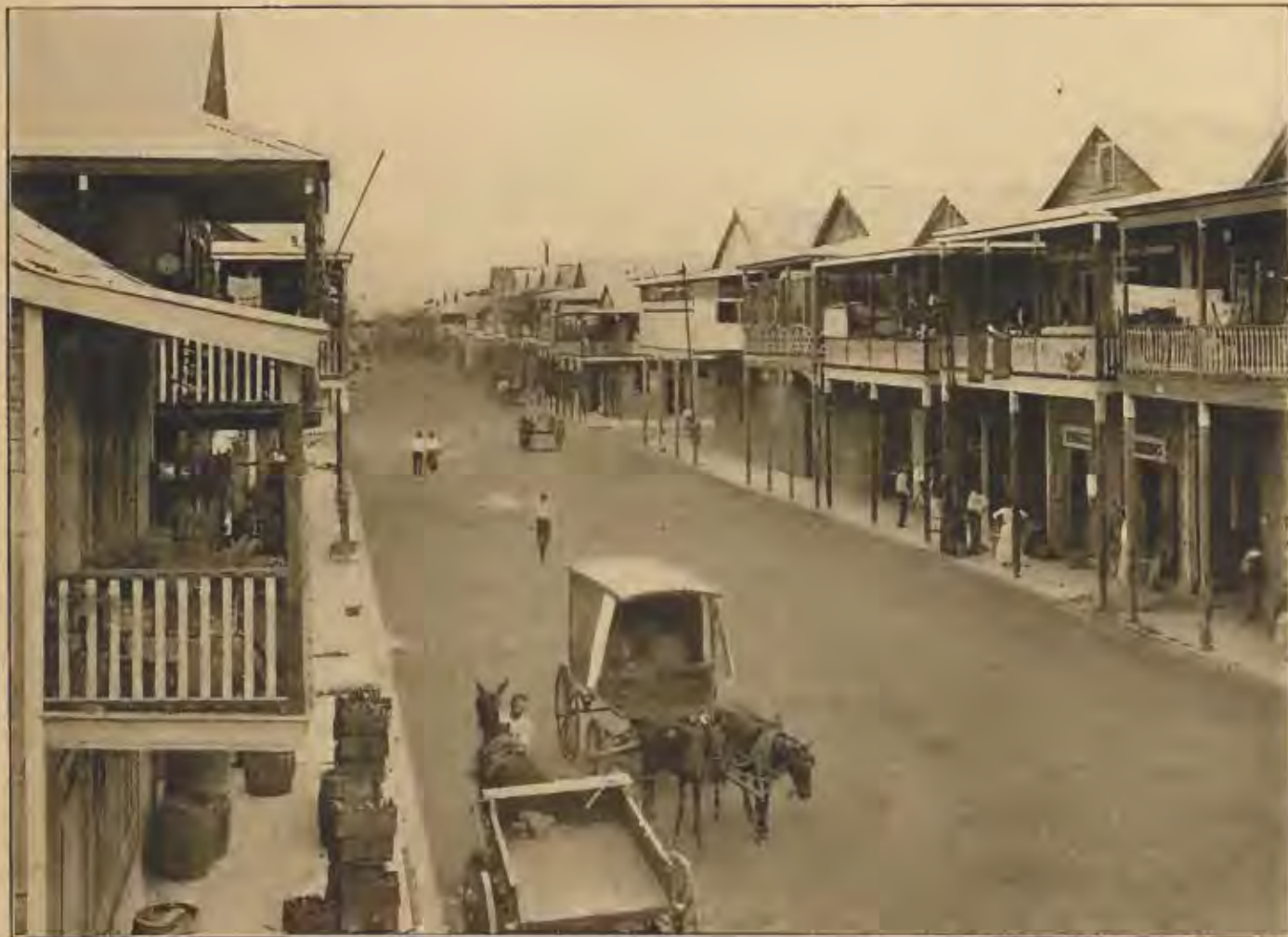
D STREET, COLON, PAVED
