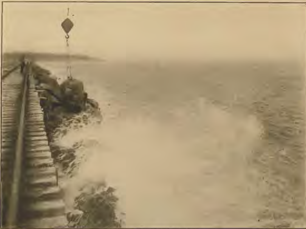
TORO POINT BREAKWATER
