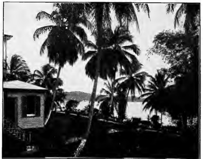
SANITARY OFFICE, BOCAS DEL TORO
