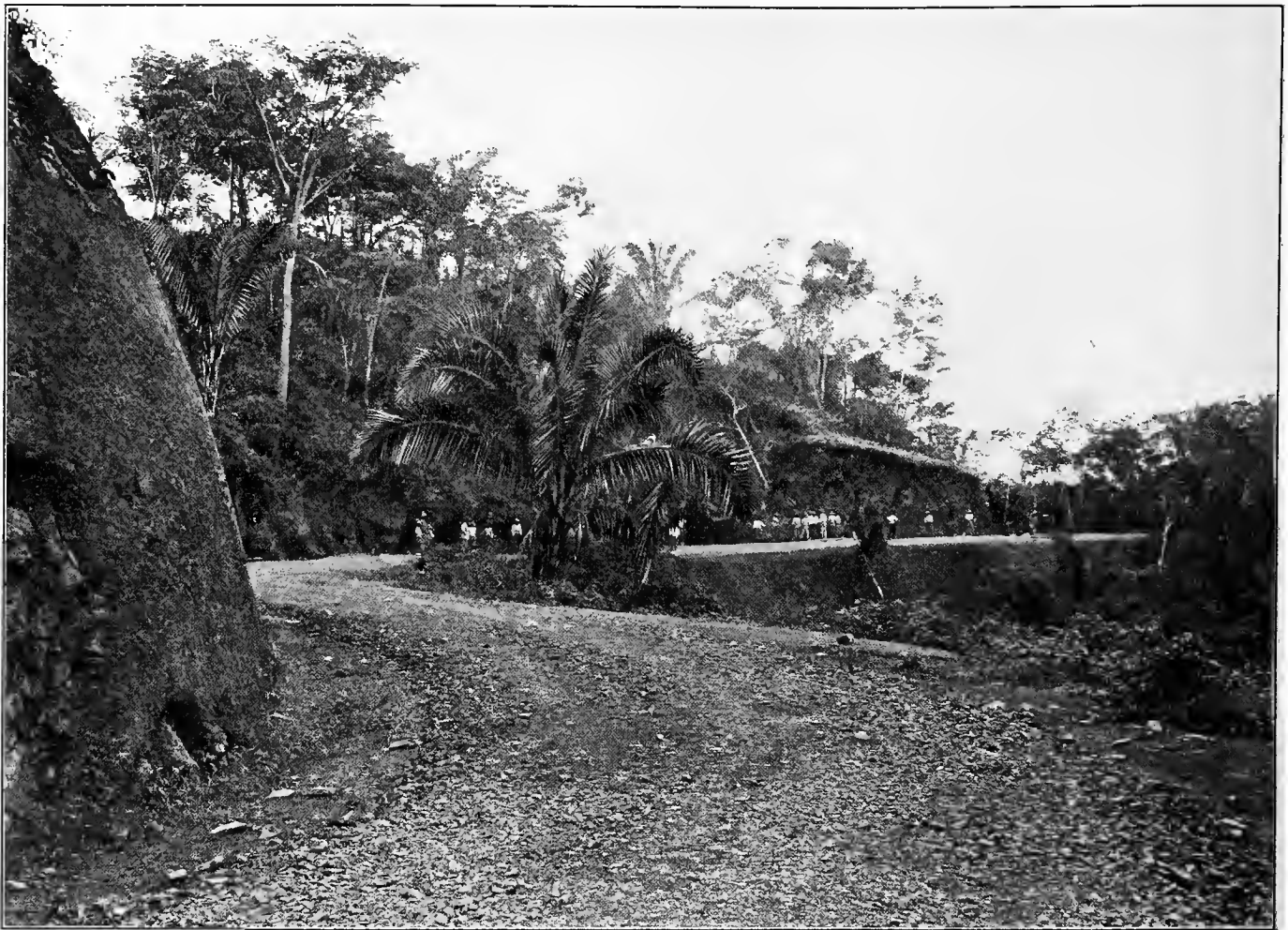
CONVICTS BUILDING A COMMISSION ROAD
