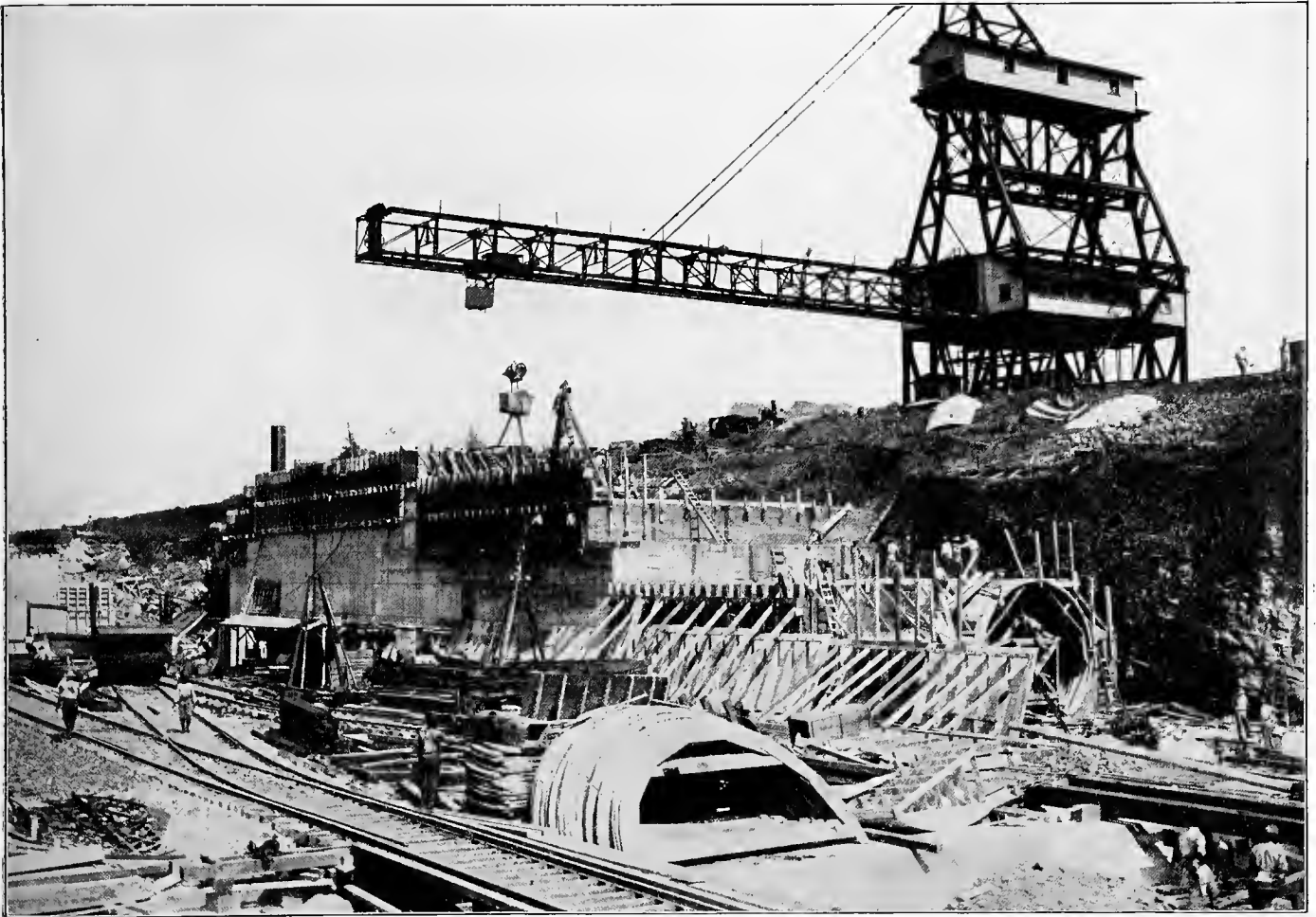
TRAVELING CRANE HANDLING CONCRETE IN LOCK-BUILDING
