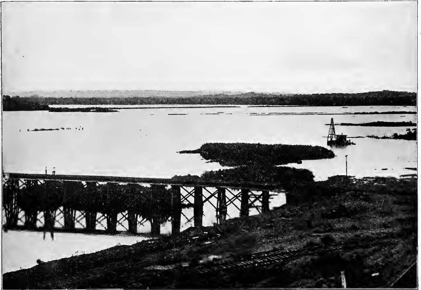
GATUN LAKE. FLOATING ISLANDS MASSED AGAINST TRESTLE
