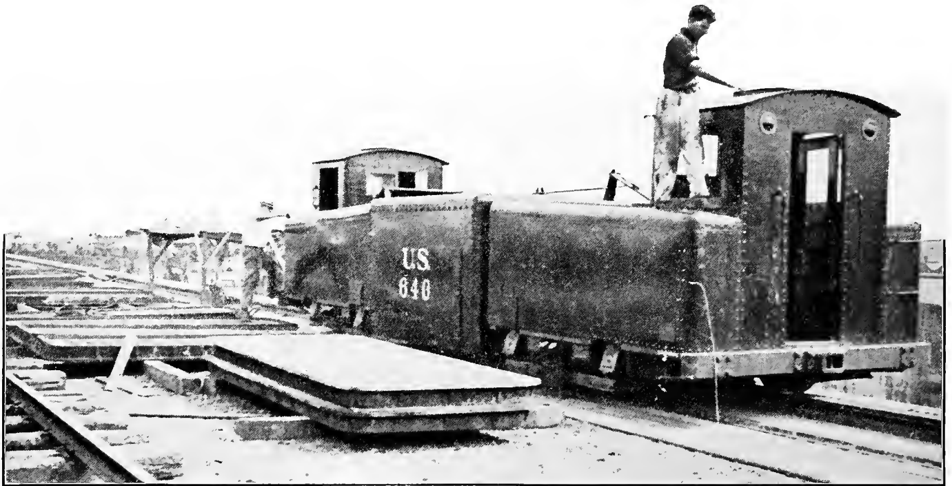
ELECTRIC TOWING LOCOMOTIVES ON A LOCK
