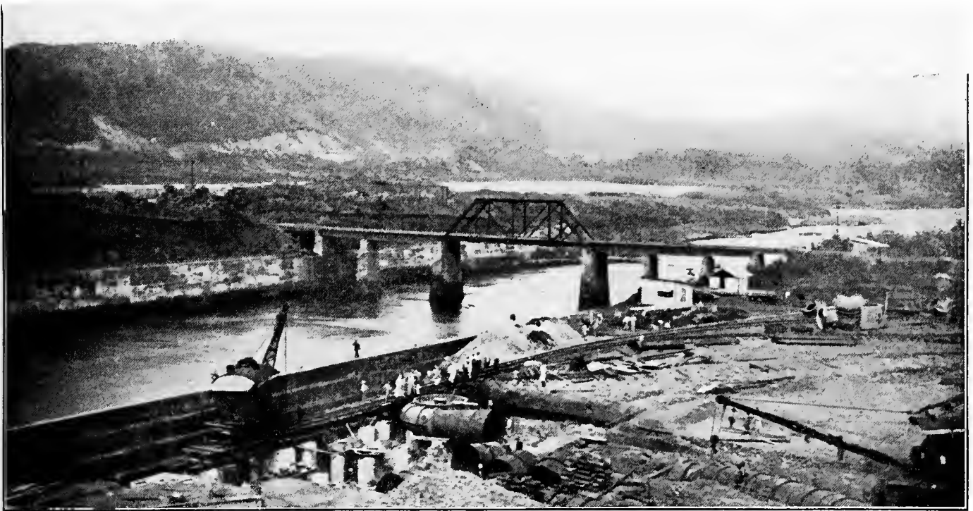
THE PANAMA RAILROAD BRIDGE AT GAMBOA
