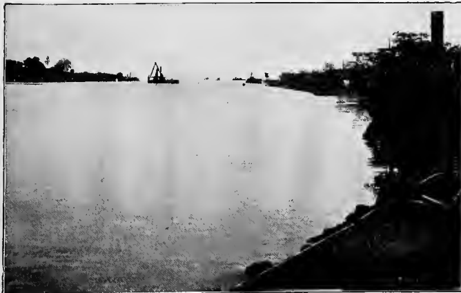
PART OF THE COMPLETED CANAL
