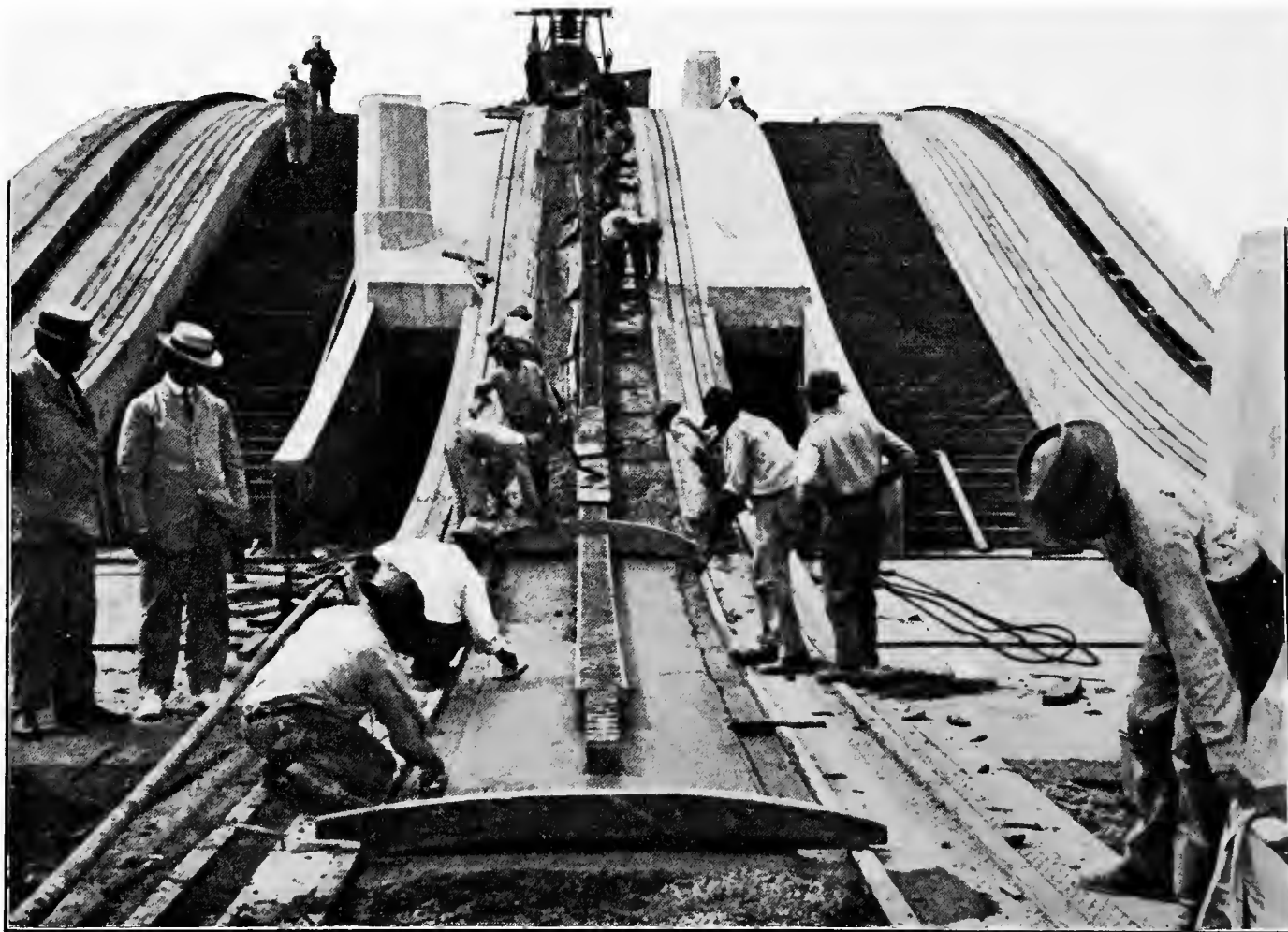
TRACKS ASCENDING FROM LOWER TO UPPER LOCK
