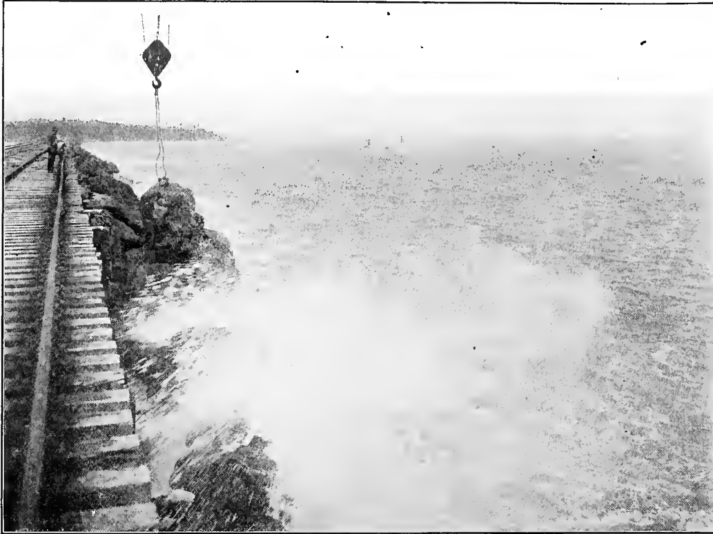
TORO POINT BREAKWATER
