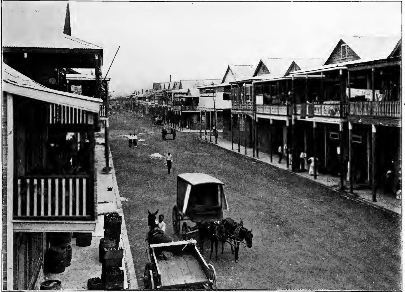
D STREET, COLON, PAVED
