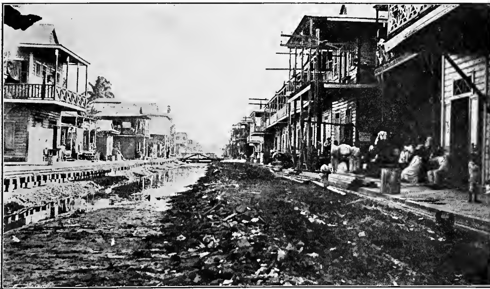
AN OPEN SEWER IN A COLON STREET
