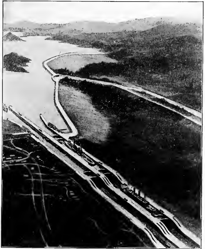
BIRD'S EYE VIEW OF GATUN DAM
