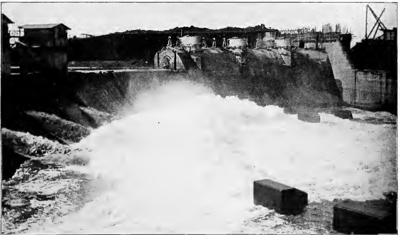
PARTLY COMPLETED SPILLWAY, 1913
