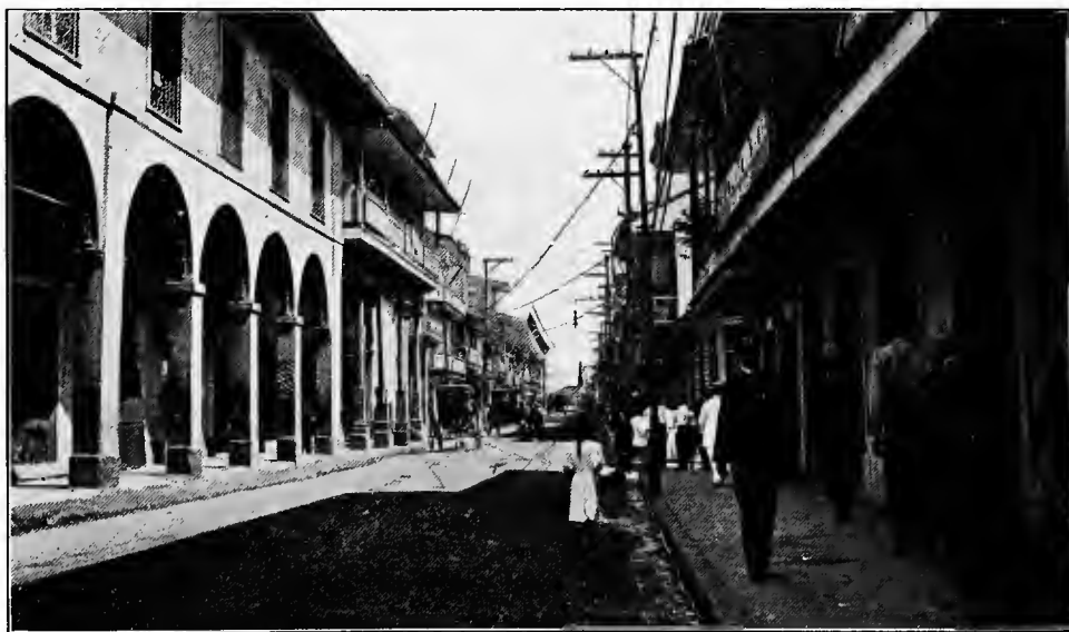
A STREET AFTER PAVING
