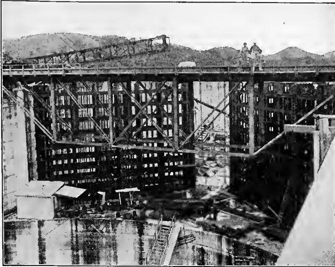
BUILDING AN UPPER TIER OF LOCKS
