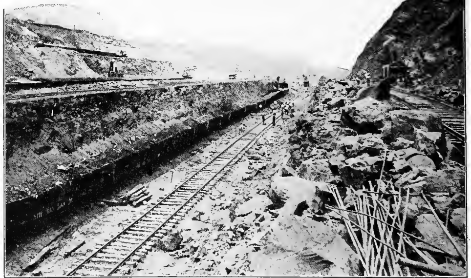
CUTTING AT BASE OF CONTRACTORS HILL
