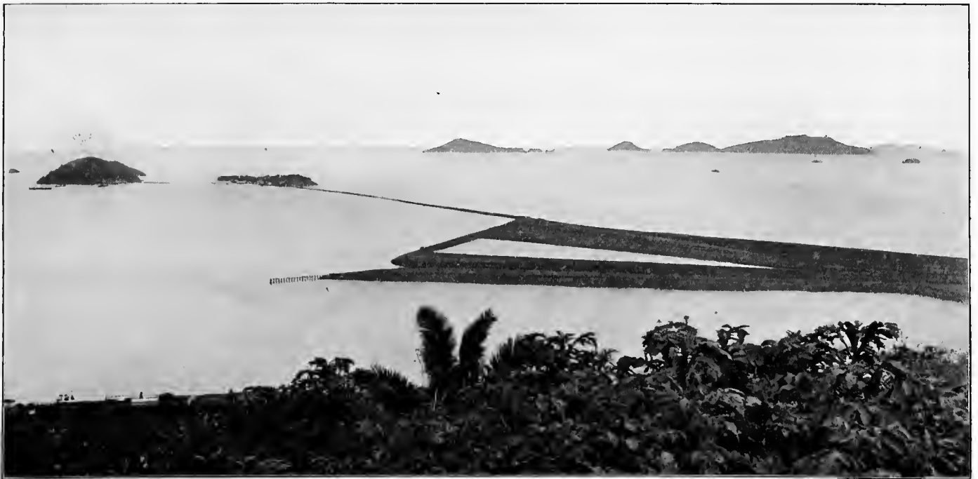
THE GREAT FILL AT BALBOA WHERE THE CULEBRA SPOIL IS DUMPED
